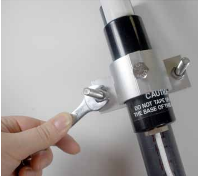
Figure 20. Mast Mount Antenna – Tighten nut on mounting bracket
