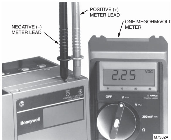
Fig. 11. Measuring flame signal voltage of 7800 SERIES controls.
