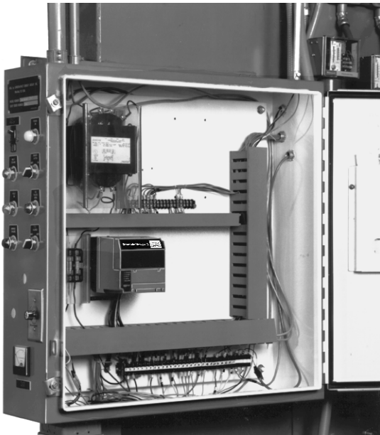
Fig. 7. Electrical panel installation.
