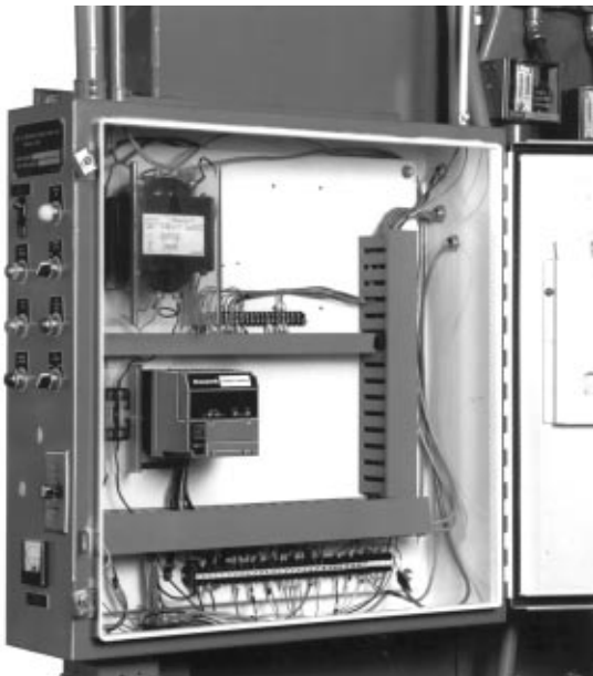
Fig. 7. Electrical panel installation.
