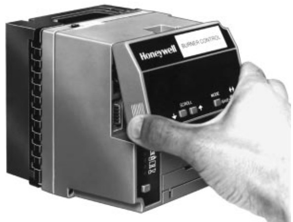
Fig. 9. Keyboard Display Module mounting.
