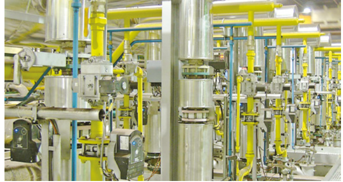
Walking beam furnace with overhead firing
