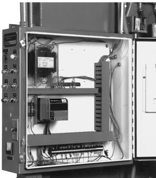
Fig. 7. Electrical panel installation.
